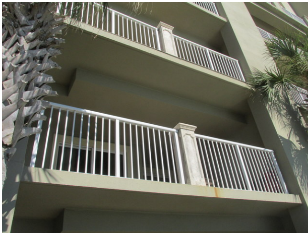
Concrete balconies and aluminum railings at Tower 1
