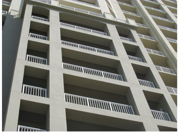
Concrete balconies and aluminum railings at Tower 1
