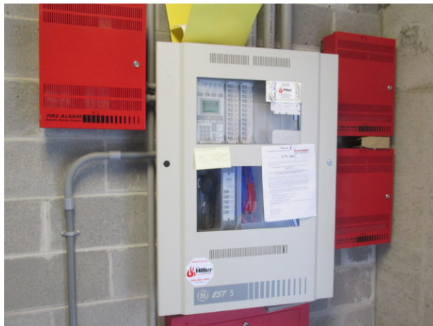
Life safety system control panel
