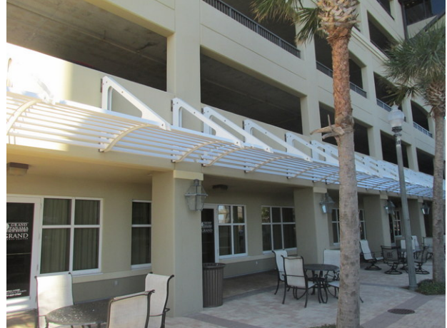
Aluminum awning at Tower 2 facade
