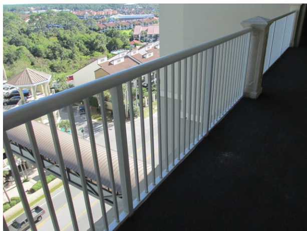
Typical aluminum railing at breezeway
