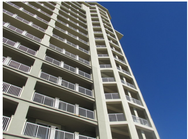
Concrete balconies and aluminum railings at Tower 2
