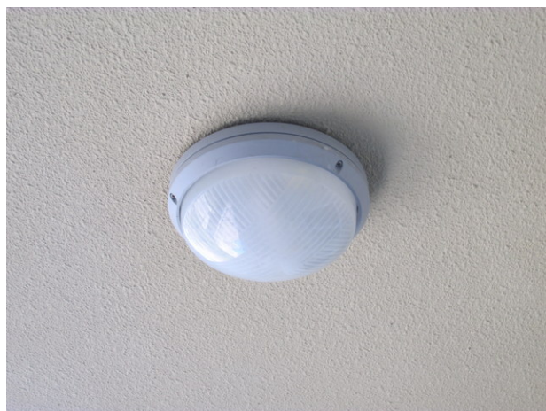
Typical ceiling-mounted breezeway light fixture
