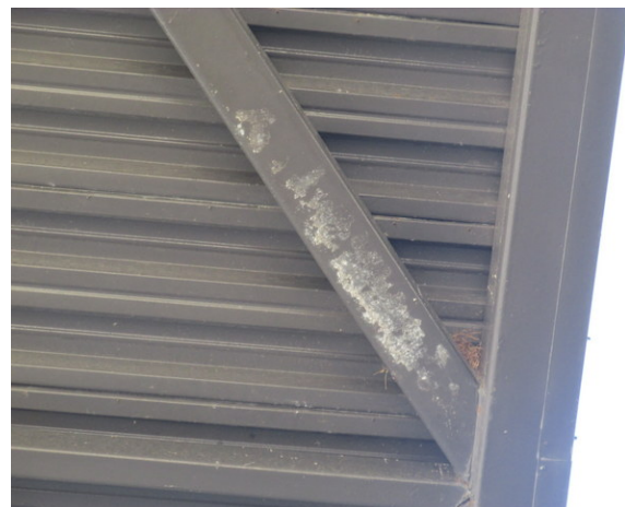
Isolated deterioration of paint finishes at skywalk
