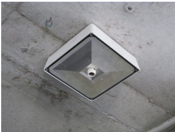
Missing bulb and cover at light fixture at separate garage structure
