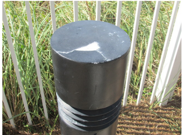
Deteriorated finishes at bollard-type light fixture at Tower 1 pool area
