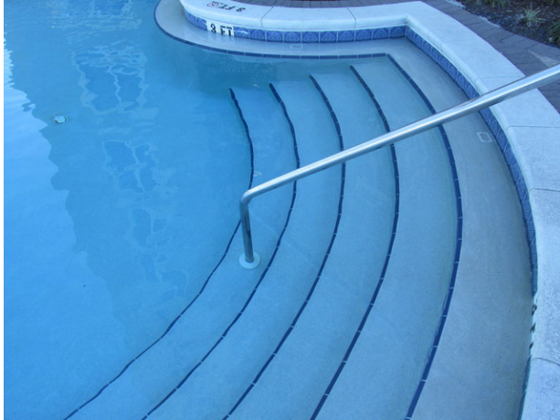
Pool plaster finish and tile at Tower 2 pool
