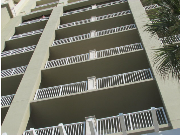
Concrete balconies and aluminum railings at Tower 1
