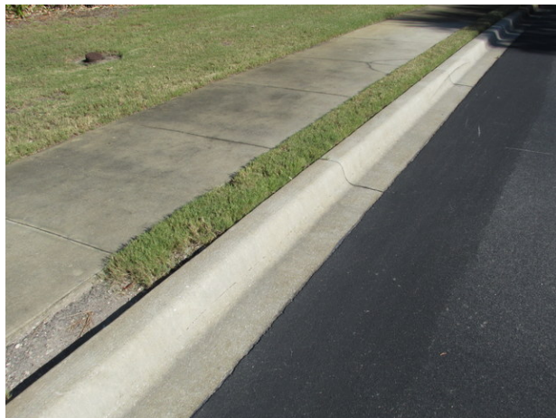
Concrete curb and gutter
