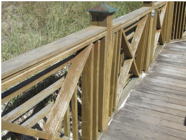
Wood decking and railings at dune walkover
