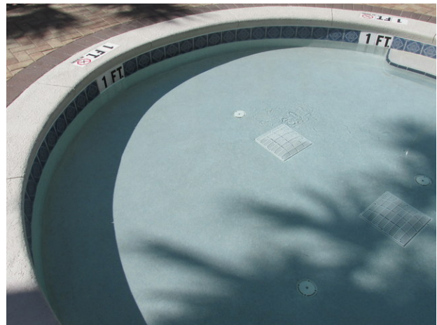
Pool plaster finish and tile at Tower 1 spa
