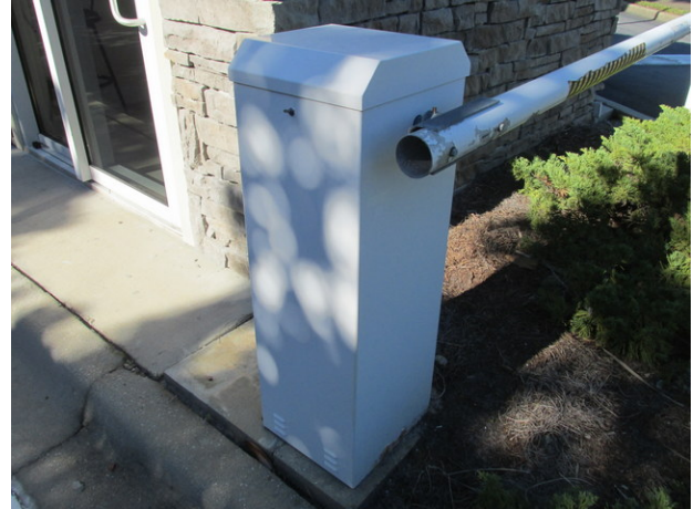
Swing-arm gate operator at gate house
