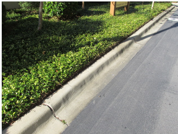
Concrete curb and gutter
