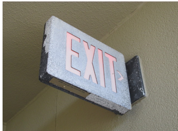
Deteriorated finishes at emergency device
