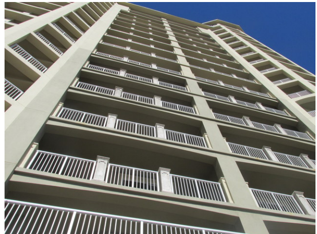
Concrete balconies and aluminum railings at Tower 2
