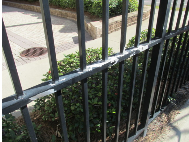
Isolated finish deterioration at aluminum fence at Tower 2 parking area
