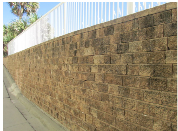
Masonry retaining wall at Tower 1 garage entrance
