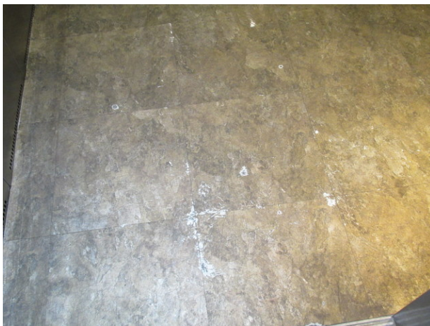
Deterioration at tile floor coverings at elevator cab
