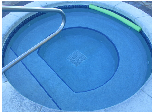
Pool plaster finish and tile at Tower 2 spa
