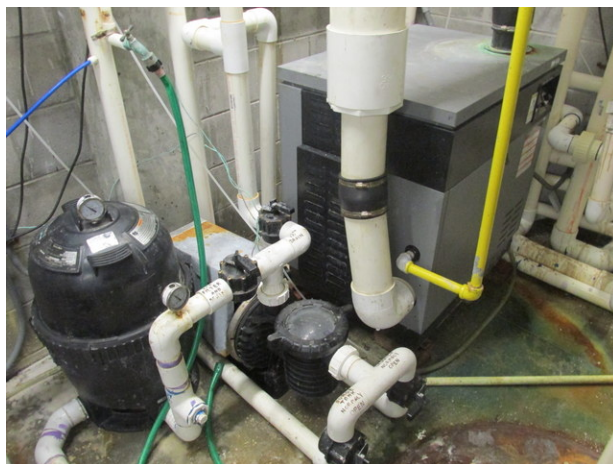
Pool mechanical equipment
