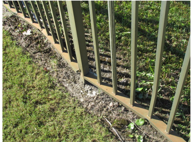
Isolated damage at aluminum fence adjacent to gate house
