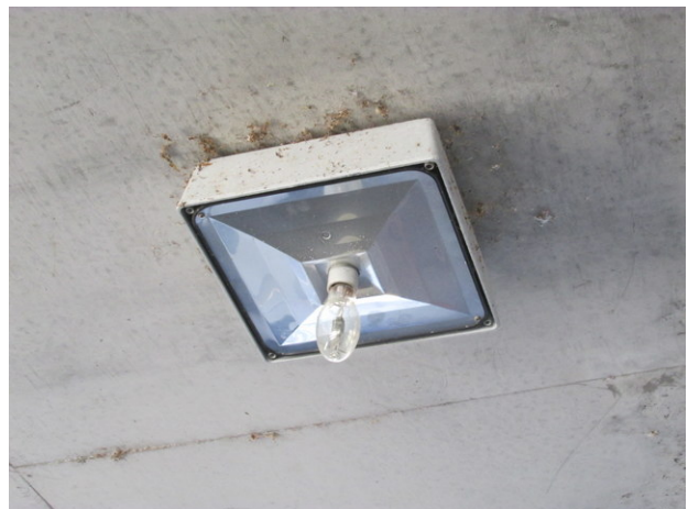
Missing cover at light fixture at separate garage structure
