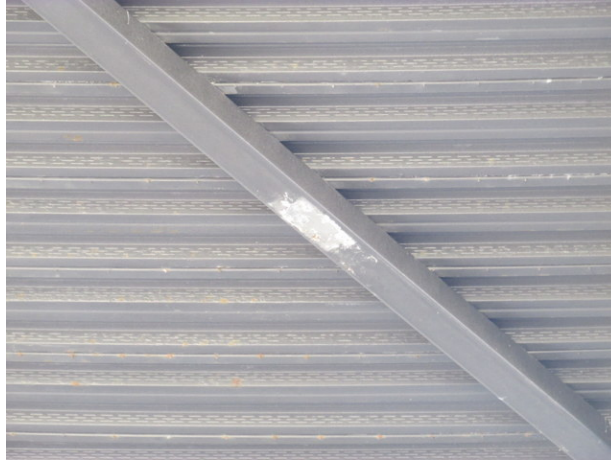
Isolated deterioration of paint finishes at skywalk
