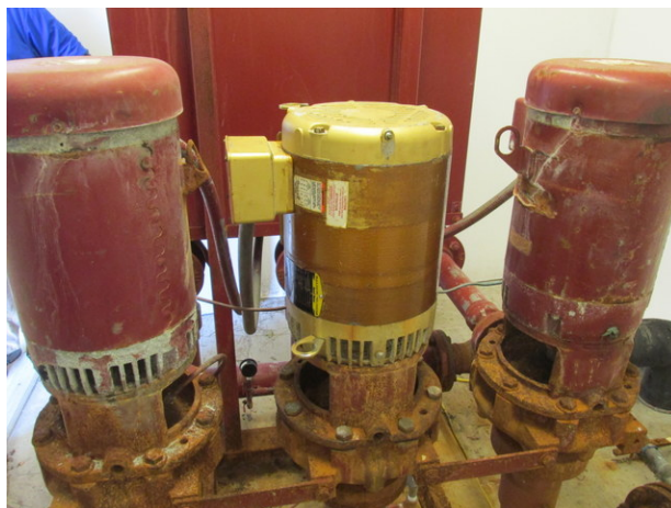
Domestic water booster pumps at Tower 1
