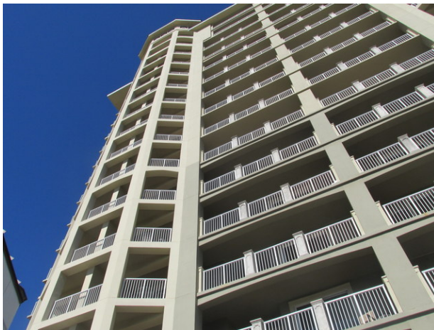
Concrete balconies and aluminum railings at Tower 2
