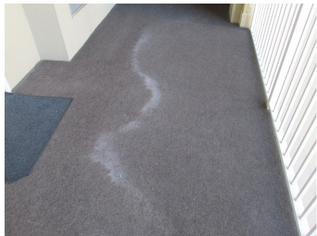
Isolated water stains at carpet floor coverings at breezeways
