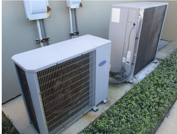
Split system condensing units
