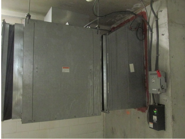
Exhaust fan at Tower 1 garage
