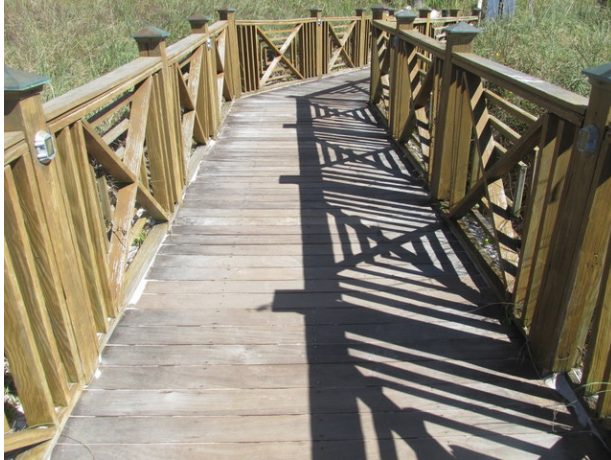
Wood decking and railings at dune walkover
