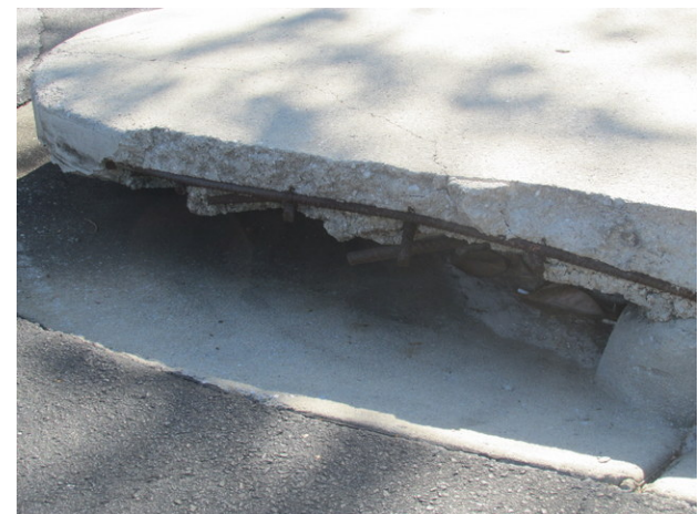
Isolated severe spalling and exposed rebar at catch basin at Tower 2 parking area
