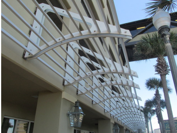
Aluminum awning at Tower 2 facade
