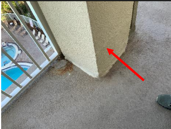
Photo 7 Unit No. 1-501 – Overall view of stucco cracking at column.
