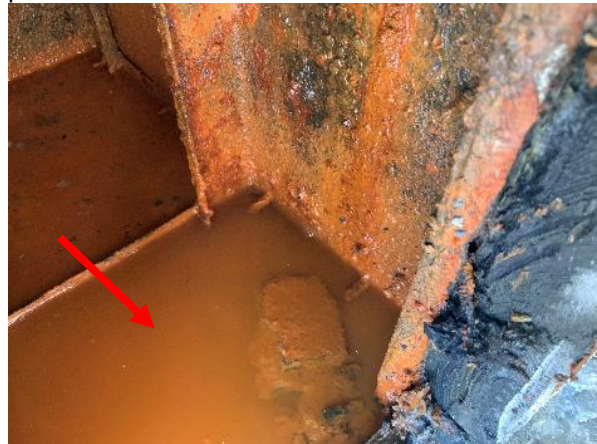
Photo 41 Tower 1 – Unit No. 1-509 – Standing water present inside of stucco column core.
