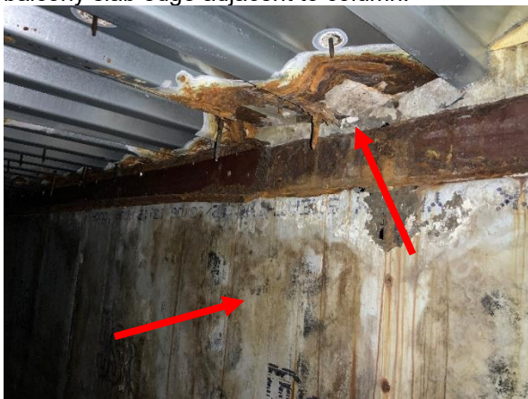
Photo 21 Column 1 – Attic Space – Overall view of deteriorated gypsum sheathing and evidence of moisture intrusion.
