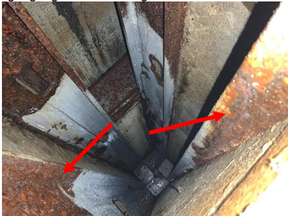
Photo 38 Unit No. 1-509 – Overall view of severely corroded light gauge metal framing members.
