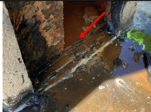
Photo 44 Unit No. 1-509 – Overall view of standing water inside column.
