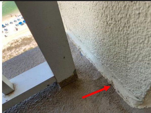
Photo 16 Unit No. 1-1201 – Microbial growth observed at column-to-deck interface.
