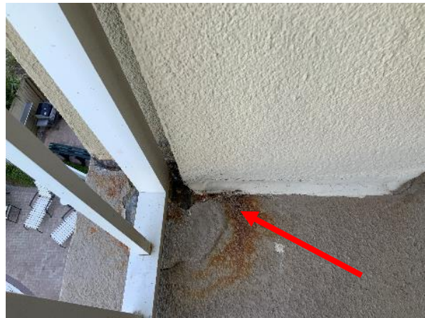
Photo 17 Unit No. 1-501 – Overall view of severe staining at balcony deck adjacent to column.
