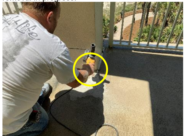
Photo 30 Tower 1 – Unit No. 1-509 – Destructive core removal in progress.
