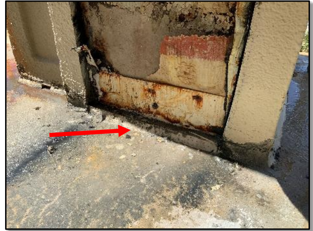
Figure 2.5.2 – Overall view of base-of-column flashing set in sealant.
