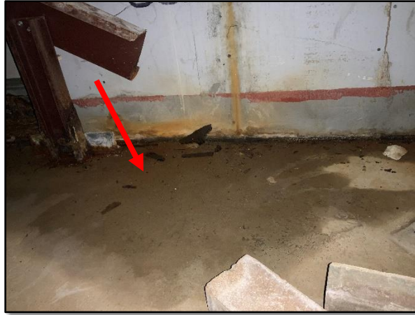
Figure 2.4.1 – Attic Space above Column 1 – Overall view of saturated concrete deck.
