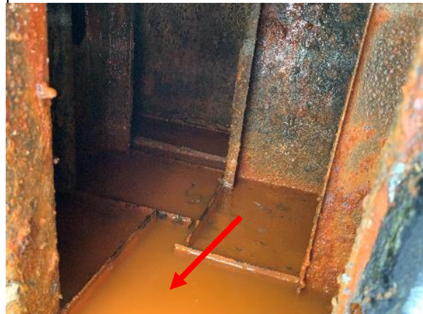
Photo 42 Tower 1 – Unit No. 1-509 – Standing water present inside of stucco column core.
