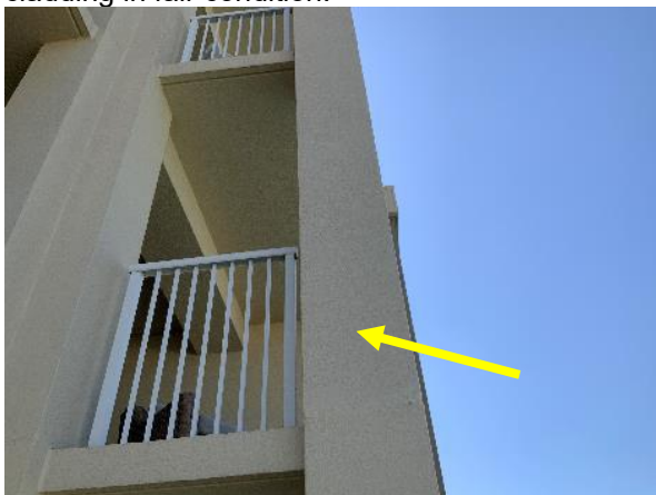
Photo 9 Tower 1 – Column No. 1 – Overall view of stucco cladding in fair condition.
