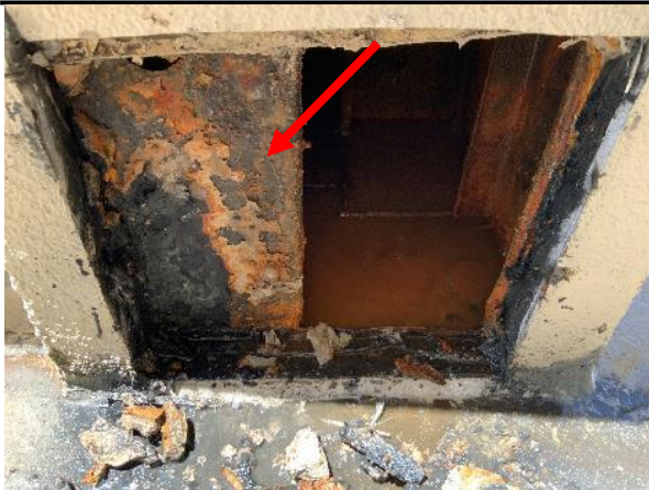
Photo 37 Unit No. 1-509 – Overall view of severely corroded light gauge metal framing members.
