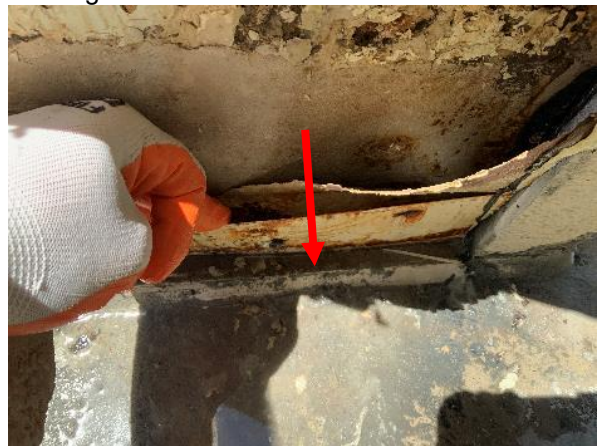
Photo 35 Unit No. 1-509 – Overall view of base of wall flashing installed on bed of sealant.
