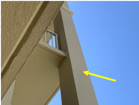
Photo 8 Tower 1 – Column No. 1 – Overall view of stucco cladding in fair condition.
