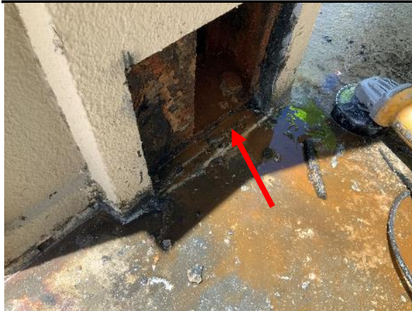
Photo 43 Unit No. 1-509 – Overall view of standing water inside column.
