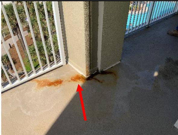
Photo 19 Unit No. 1-509 – Overall view of severe staining at balcony deck adjacent to column.
