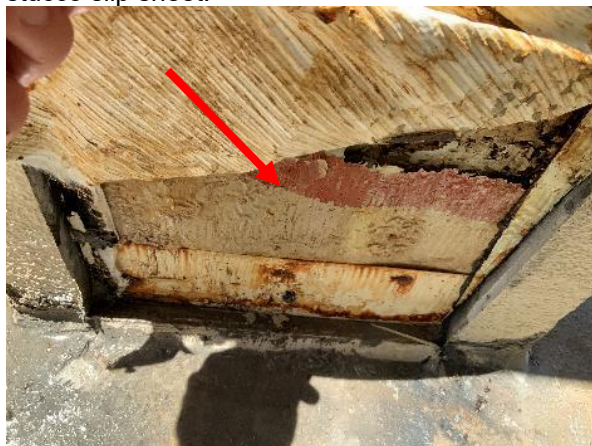
Photo 33 Unit No. 1-509 – Overall view of self-adhered flashing behind base-of-column flashing.
