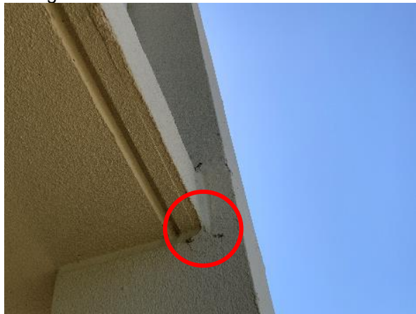
Photo 14 Unit No. 1-509 – Overall view of microbial growth at column-to-ceiling interface.
