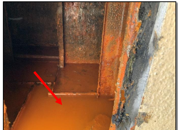
Figure 2.5.4 – Overall view of standing water in base-of-column condition.
