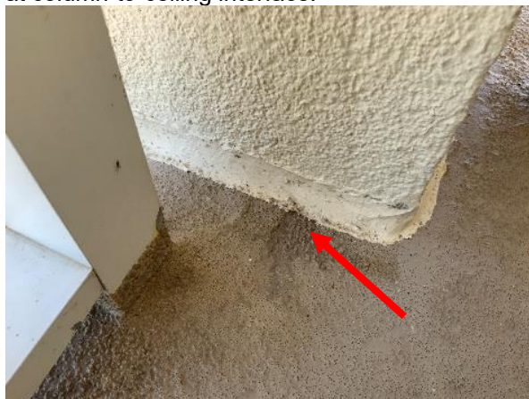
Photo 15 Unit No. 1-1201 – Microbial growth observed at column-to-deck interface.
