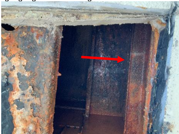
Photo 39 Unit No. 1-509 – Overall view of severely corroded light gauge metal framing members.
