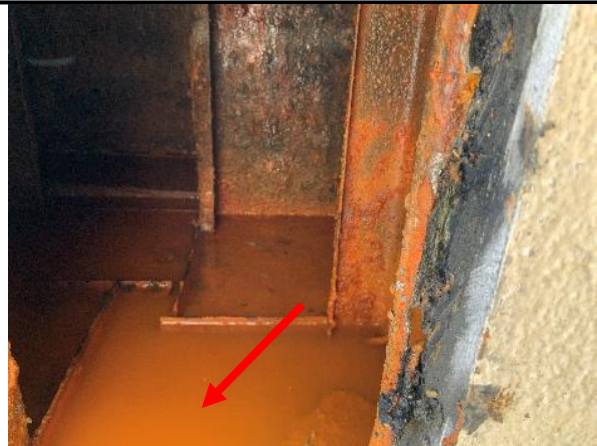
Photo 40 Tower 1 – Unit No. 1-509 – Standing water present inside of stucco column core.
