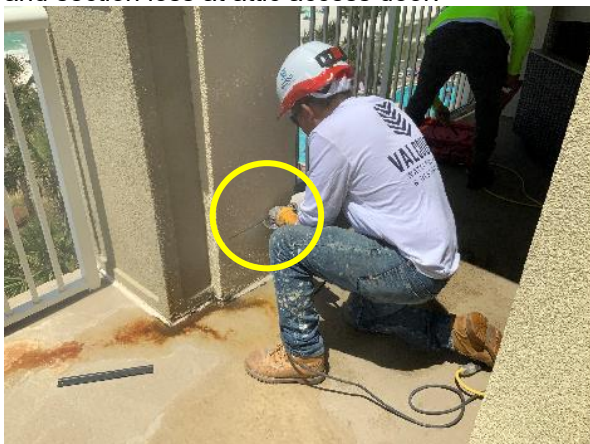
Photo 27 Unit No. 1-509 – Overall view of core removal in progress.
