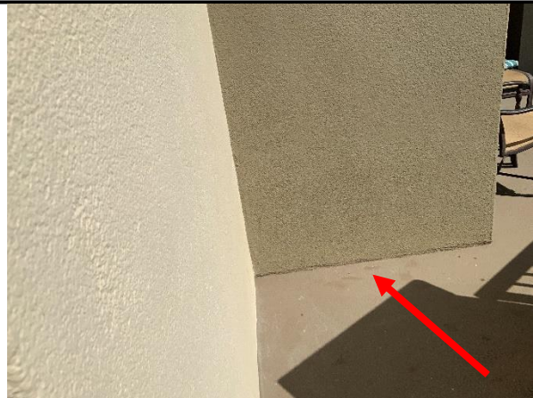
Photo 4 Tower 2 – Column 8 – Overall view of column sealed at base-of-wall condition.
