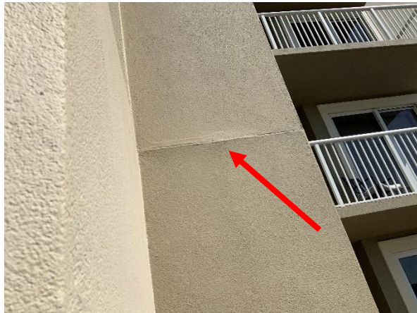
Photo 2 Tower 2 – Column 8 – Overall view of delaminated stucco cladding at floor line.
