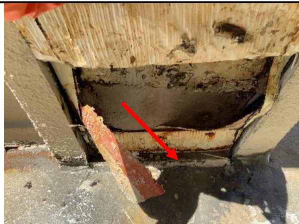
Photo 34 Unit No. 1-509 – Overall view of base of wall flashing installed on bed of sealant.
