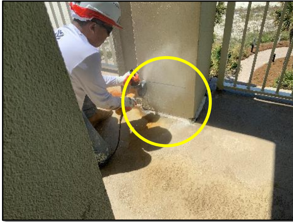
Figure 2.5.1 – Stucco core removal in progress.
