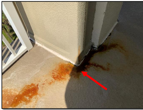
Figure 2.3.1 – Unit No. 1-509, Column 9 – Overall view of staining at deck.
