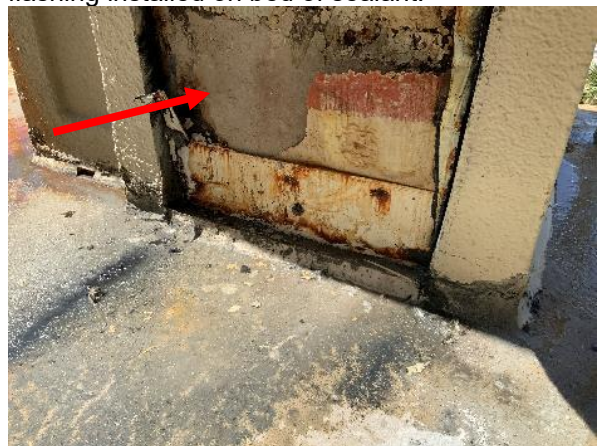
Photo 36 Unit No. 1-509 – Overall view of saturated and deteriorated gypsum sheathing.
