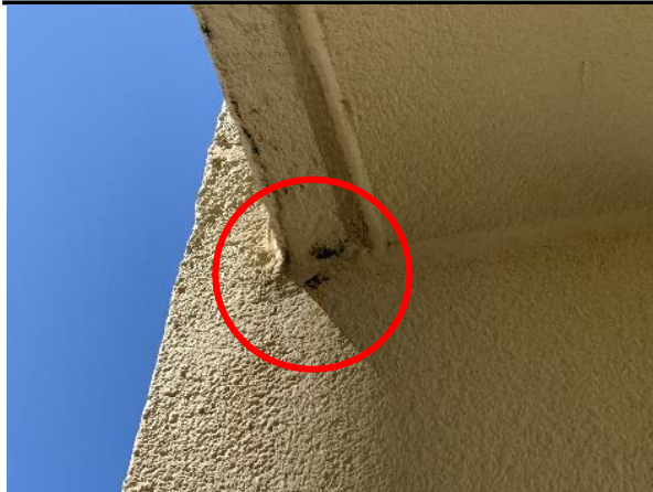
Photo 13 Unit No. 1-1209 – Overall view of coating failure and microbial growth observed at column-to-ceiling interface.
