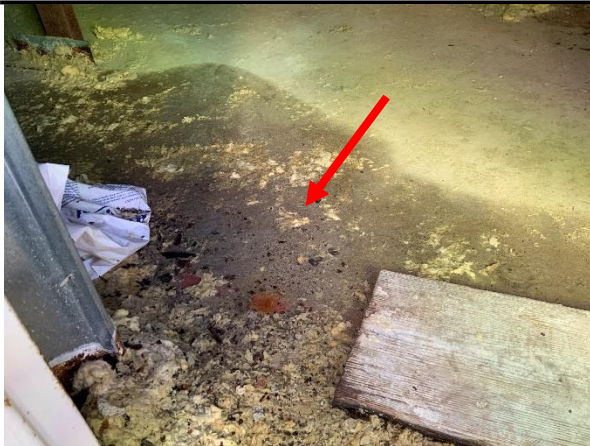
Photo 25 Column 9 – Attic Space – Overall view of saturated concrete deck.
