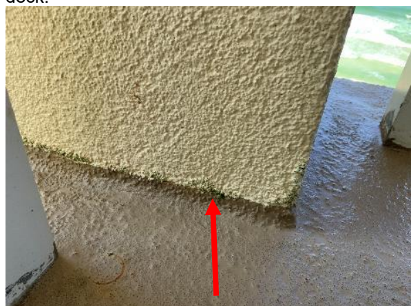
Photo 12 Unit No. 1-1209 – Overall view of microbial growth at base-of-column.
