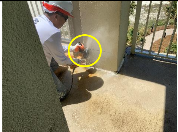
Photo 28 Tower 1 – Unit No. 1-509 – Destructive core removal in progress.
