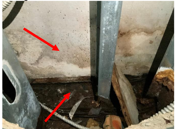
Photo 23 Column 9 – Attic Space – Overall view of corroded framing track and saturated sheathing.
