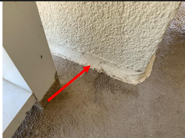
Photo 10 Unit No. 1-1201 – Overall view of column sealed to deck.
