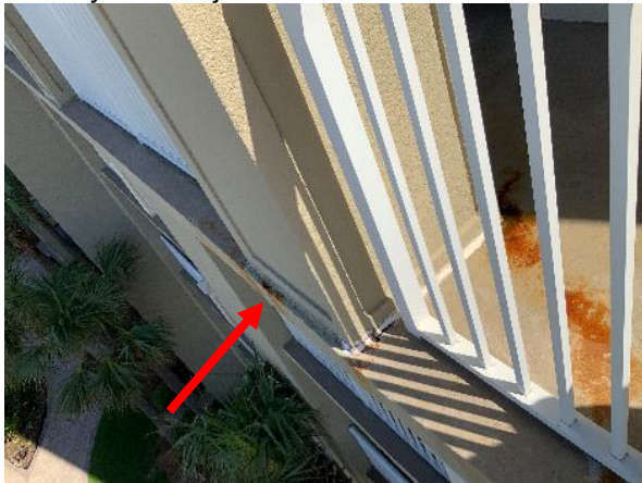
Photo 20 Unit No. 1-509 – Overall view of staining at balcony slab edge adjacent to column.
