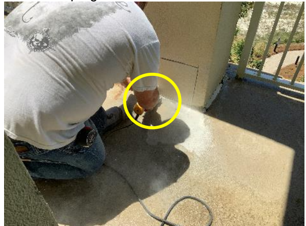
Photo 29 Tower 1 – Unit No. 1-509 – Destructive core removal in progress.
