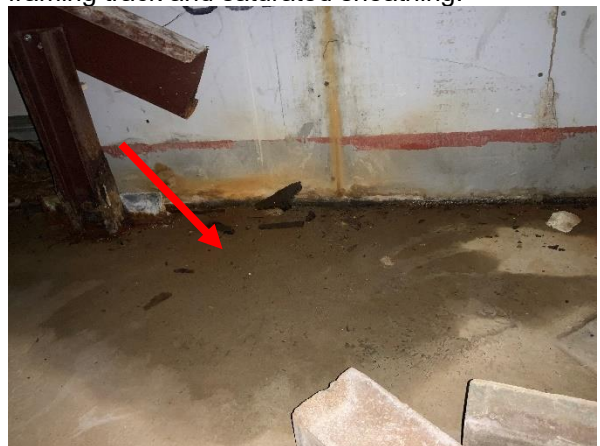
Photo 24 Column 1 – Attic Space – Overall view of saturated concrete deck.
