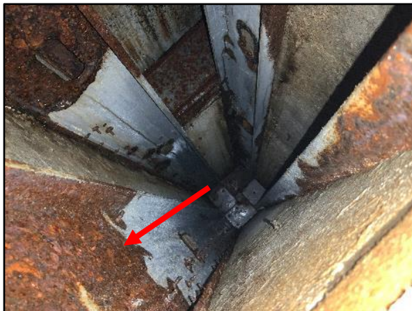
Figure 2.5.3 – Overall view of severely deteriorated light gauge metal framing.
