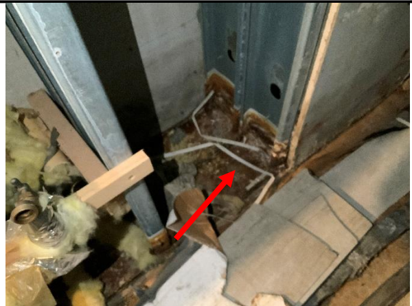
Photo 22 Column 1 – Attic Space – Overall view of corroded framing track.
