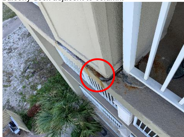
Photo 18 Unit No. 1-501 – Overall view of severe staining at balcony deck adjacent to column.
