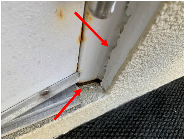
Photo 26 Unit No. 1-2109 – Overall view of severe corrosion and section loss at attic access door.
