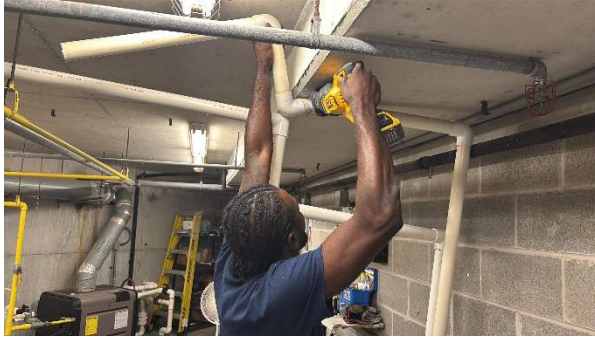
Repairs to pool plumbing line
