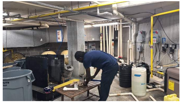
Repairs to pool plumbing line
