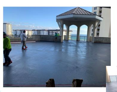
Level 5 deck coating is complete, waiting for traffic striping
