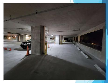
Level 2 - Phase 2 (Outside half), shotblast completed ready for traffic coating.
