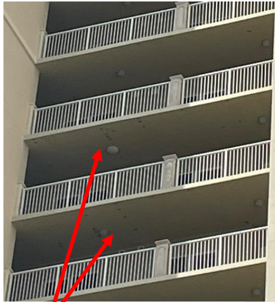
Rust Spot Repairs
