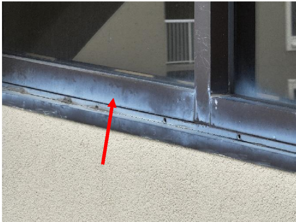
Photo 25 Window Assemblies – Overall view of faded finish and oxidation at the window sill frame and flashing.
