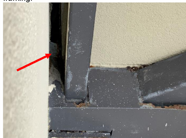
Photo 30 Skybridge-to-Garage Interface – West Elevation – Overall view of missing sealant and exposed framing.
