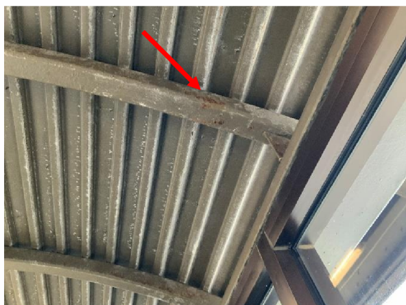
Photo 7 Interior – Overall view of corrosion at roof purlin.
