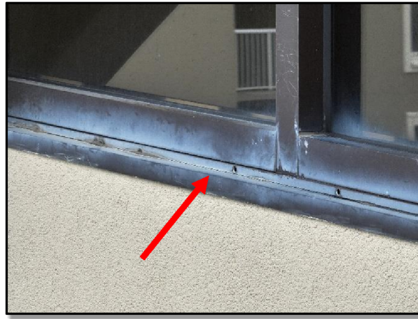
Figure 2.6.1 – Overall view of faded coatings and oxidation at window sill frame and flashing.
