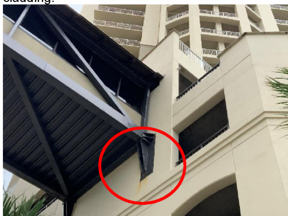
Photo 21 North Elevation – Overall view of staining at the stucco cladding beneath the Skybridge attachment bracket.
