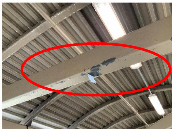
Photo 10 Interior – Overall view of failed coatings at steel beam.
