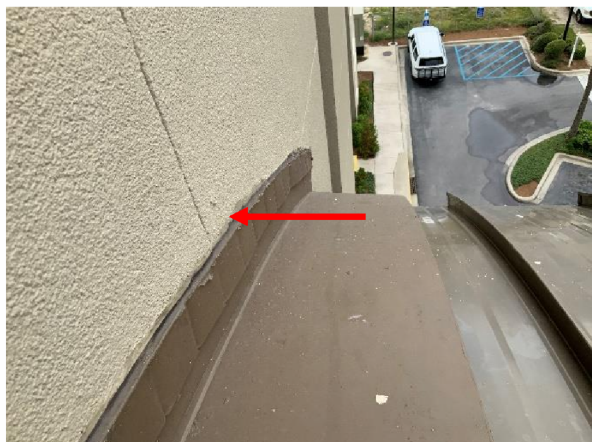
Photo 19 South Elevation – Overall view of the headwall flashing sealed to the conventional stucco cladding.
