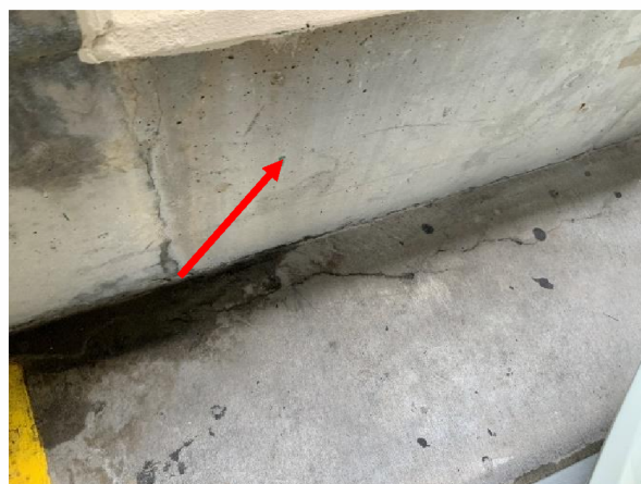
Photo 24 Parking Garage – Overall view of cracked and unsealed concrete knee wall.
