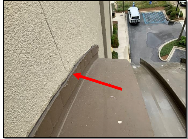
Figure 2.4.2 – Close-up view of headwall flashing sealed to conventional stucco cladding.
