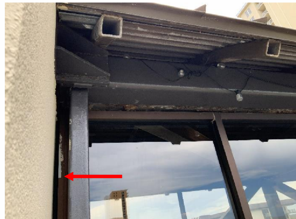
Photo 29 Skybridge-to-Garage Interface – West Elevation – Overall view of missing sealant and exposed framing.
