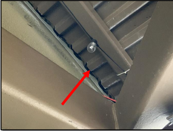
Figure 2.4.1 – Close-up view of roofing underlayment terminated at end of steel roof deck.
