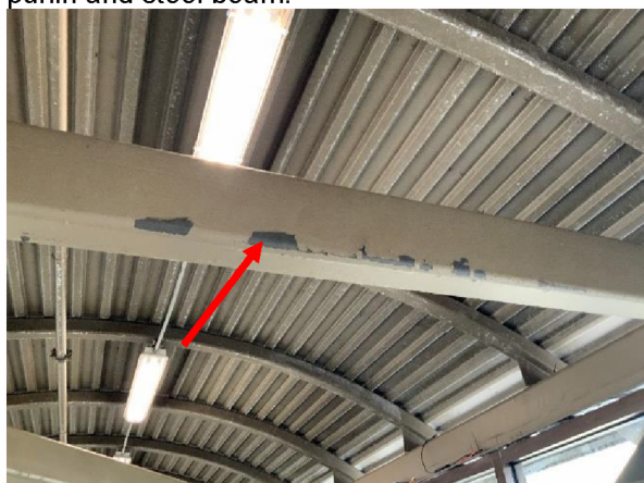
Photo 9 Interior – Overall view of failed coatings at steel beam.
