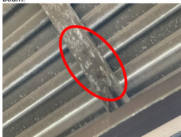
Photo 11 Interior – Overall view of failed coatings and corrosion at roof purlin.
