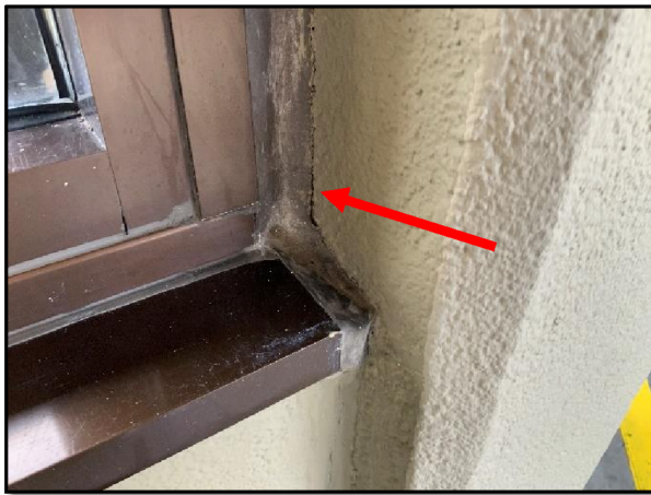
Figure 2.7.1 – Close-up view of isolated area of failed sealant at North expansion joint.
