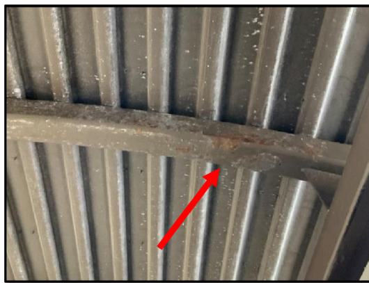
Figure 2.2.1 – Close-up view of failed coating and corrosion at steel roof purlin.
