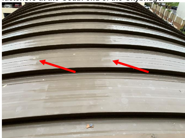
Photo 15 Roof – Overall view impact damage to the roof panels.
