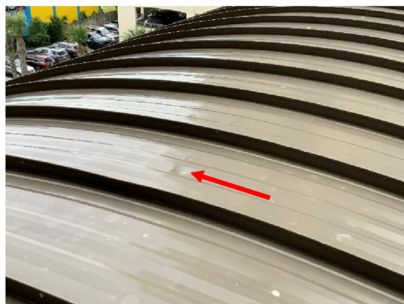
Photo 16 Roof – Overall view impact damage to the roof panels.
