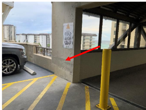
Photo 22 Parking Garage – Overall view of unsealed concrete adjacent to the stained stucco cladding.
