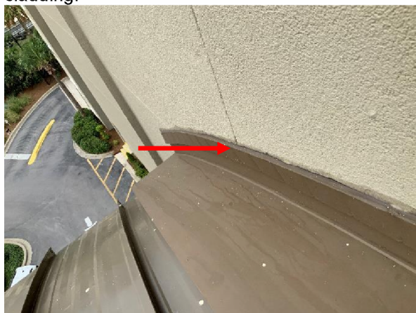
Photo 20 South Elevation – Overall view of the headwall flashing sealed to the conventional stucco cladding.
