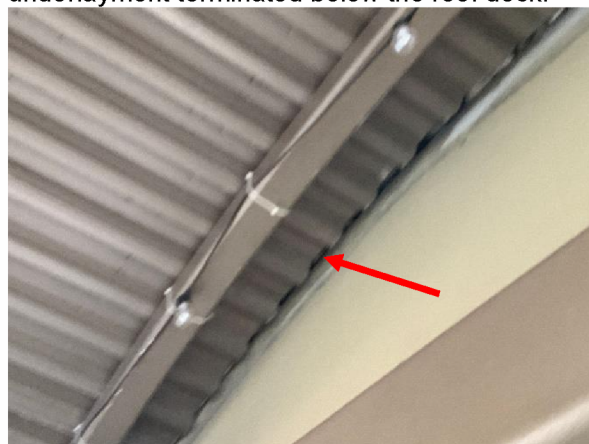
Photo 18 South Elevation – Overall view of the roofing underlayment terminated below the roof deck.
