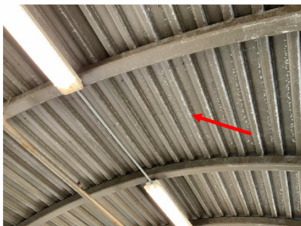
Photo 13 Interior – Overall view of failed coatings at the steel roof deck.
