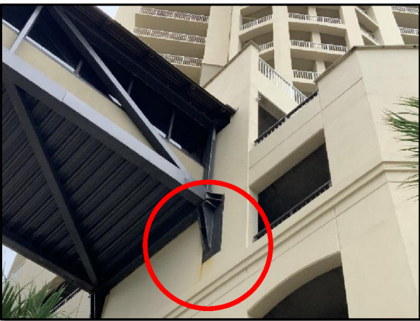
Figure 2.5.1 – Overall view of staining at stucco cladding below Skybridge attachment bracket.
