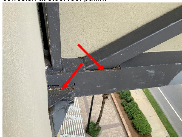
Photo 6 West Elevation – Overall view of corroded attachment brackets and framing members.
