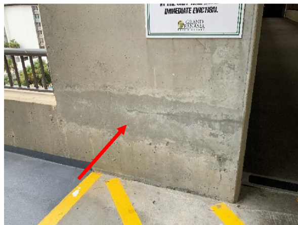
Photo 23 Parking Garage – Overall view of cracked and unsealed concrete column.
