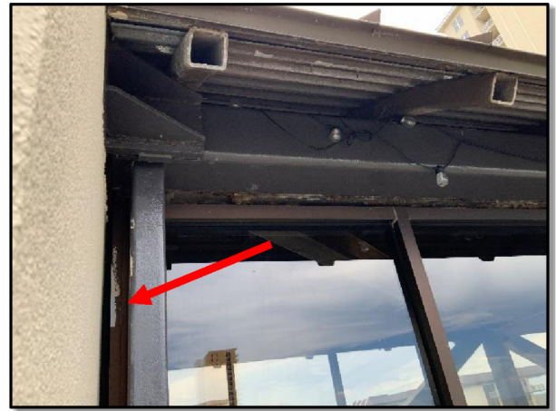
Figure 2.7.1 – Close-up view of missing sealant at Skybridge-to-Parking Garage interface.
