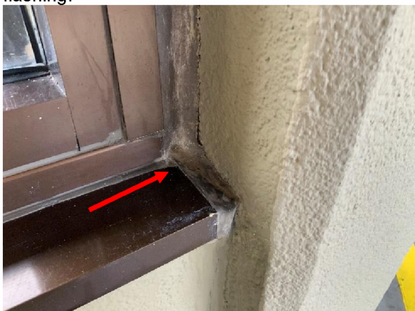
Photo 27 North Entrance – Overall view of isolated failed sealant at the expansion joint.
