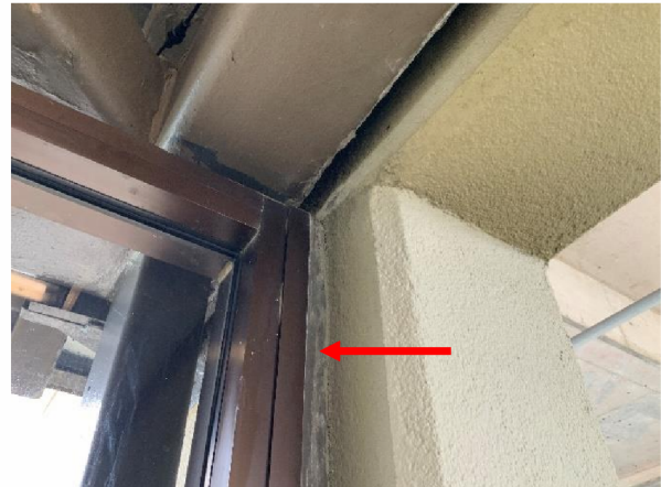
Photo 28 North Entrance – Overall view of isolated failed sealant at the expansion joint.
