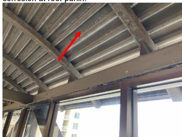
Photo 12 Interior – Overall view of failed coatings at the steel roof deck.
