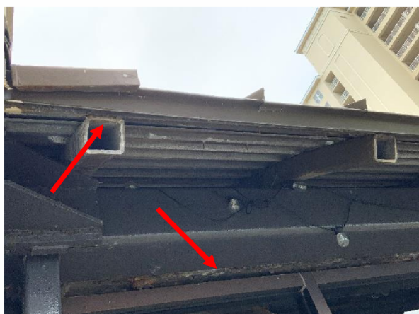
Photo 8 West Elevation – Overall view of corrosion at roof purlin and steel beam.
