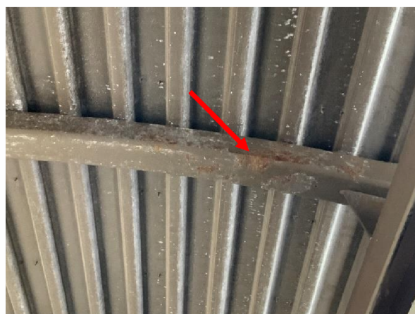
Photo 5 Interior – Close-up view of failed coating and corrosion at steel roof purlin.
