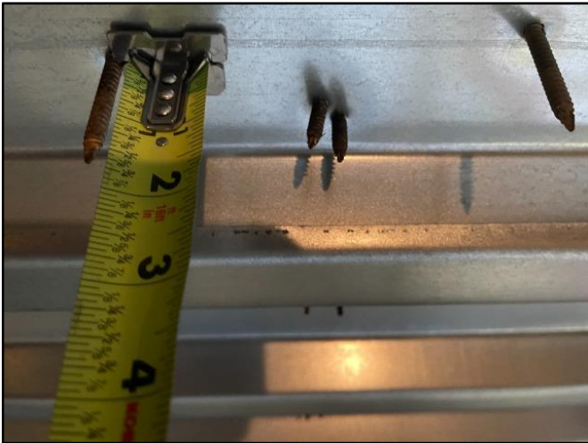
Roof Sheathing Nail Size
