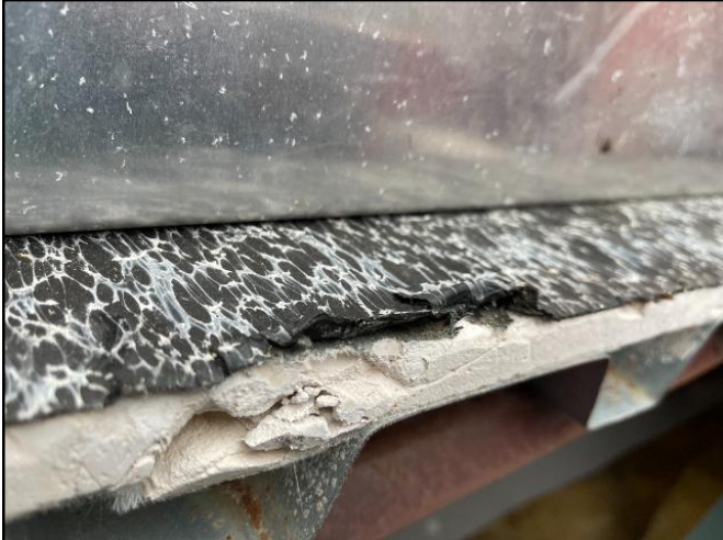
SWR (Secondary water resistant layer)
