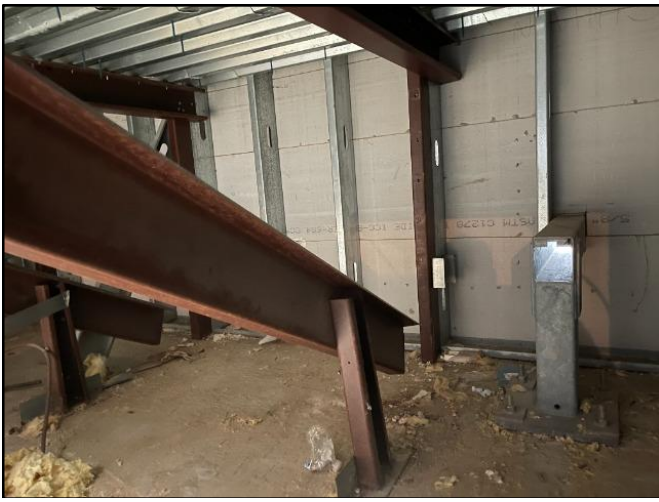
Roof to Wall Attachment
